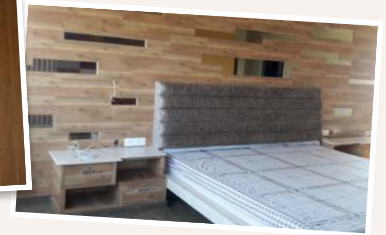
Flooring used in Wall Paneling in Hotel Room
